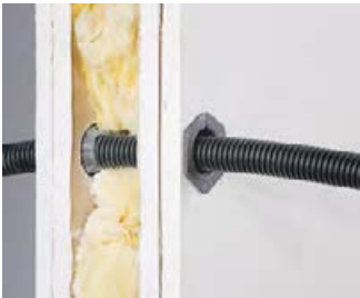
Wall feed-through in plasterboard fire-protection wall.
