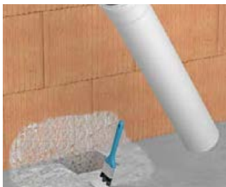
Pre-treat mineral bases and fibreboards with primer.
