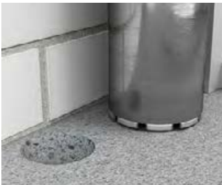
Making a core drill hole 150 mm or 100 mm.
