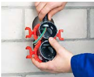
Creating installation opening.
