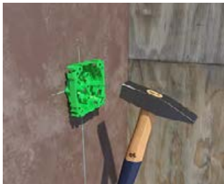
Fix the front part to the working formwork.
