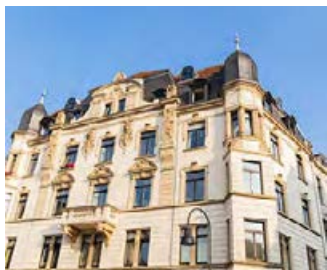
Historically significant facades in exposed masonry or stucco facades.
