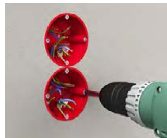
Fixing the boxes in the installation opening.
