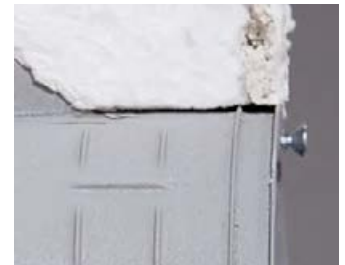
The all-round sealing lip seals the EIFS, so no moisture can penetrate.
