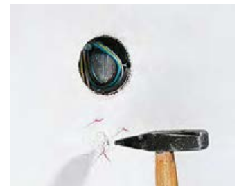
Fine marker bristles on the signal cover show the exact position of the one-gang box after plastering.
