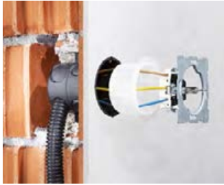
Later air-tight closing of flush-mounting boxes.
