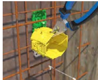
Open the conduit entry.
