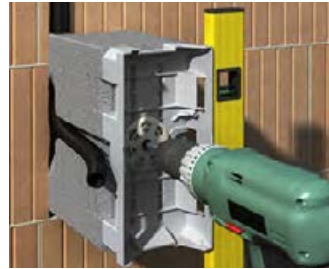
Hold the equipment carrier against the wall, align it, and fix it using the dowel.
