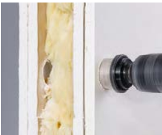
Cut a 35 mm installation opening using e.g. the KAISER MULTI 4000 cutter (Art. No. 1082-10).
