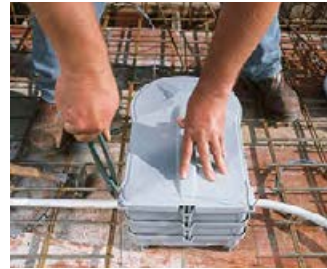
Also secure the housing to the reinforcement.
