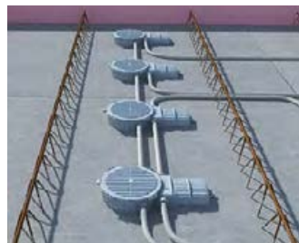
After fitting of the conduits, concreting on the planned ceiling thickness takes place with the on-site mixed concrete process.
