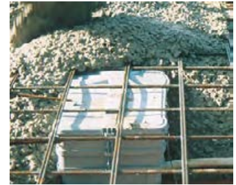
Secure and firm seating of housings during concreting.
