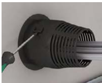
Loosen the sealing element by turning it a quarter of a turn and open it.
