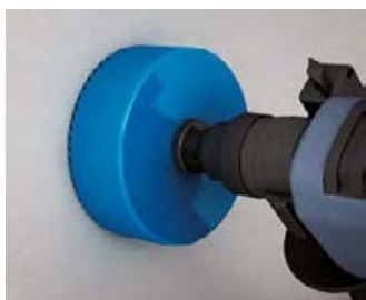
Cut installation opening with a cutter Ø 120 mm (e.g. bi-metal-cutter Art. No. 1082-20).
