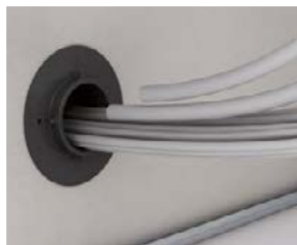
Insert the new cables and conduits.
