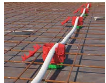
The advantage of the new cable entry is that inserting empty conduits for multiple ceiling junction boxes in one line can take place by simple laying of the installation conduit without cutting it before.
