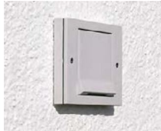
Accessory installation without disrupting the insulation or creating heat bridges.
