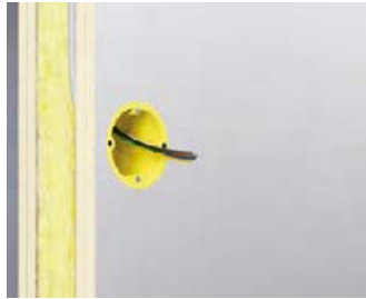
Installation of the radiation protection box in the wall.
