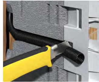
Press the conduit into the side guide and cut it to length.
