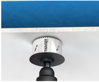
Make the cut opening.
