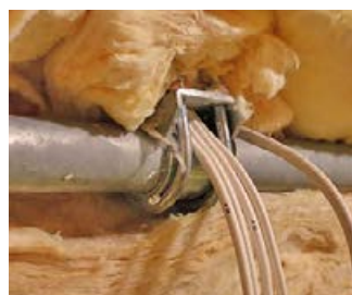
The mast which supports the parabolic mirror must also be incorporated in the equipotential bonding.
