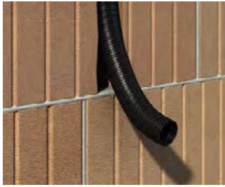
Masonry with conduit Exit.
