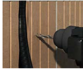
Cut Ø 8 mm drill hole at least 50 mm deep.
